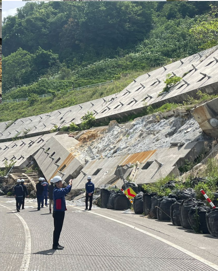
Large scale slope failure in the loop area
