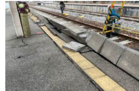
Wakura Spa St. (platform sinking etc.)
