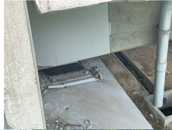
Large skidding of the pier bearing section
