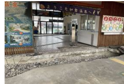
Wakura Spa St. (platform sinking etc.)
