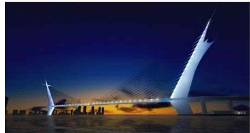
3 rd Connection Mactan - Cebu Mainland Bridge
