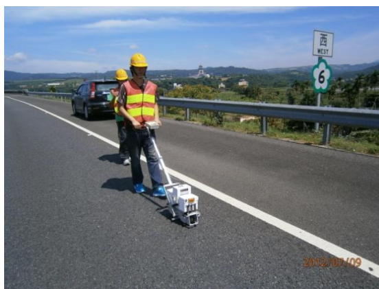
Figure 5 Measurement of pavement smoothness
