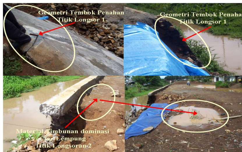
Figure 6. The construction material for pavement and protection wall at both slide spots.
