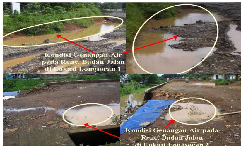
Figure 5. The pattern of failure for both slide spots, Jln. Inspeksi Saluran Air Baku PDAM Kota Makassar.
