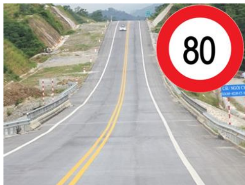
Initial-phase expressway investment includes a 2×3.5m carriageway, a 2×2m treated shoulder, and no median barrier.
