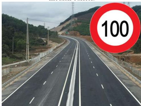
Full-phase expressway investment includes a 4×3.75m carriageway with a median barrier and 2×3m emergency stopping lanes
