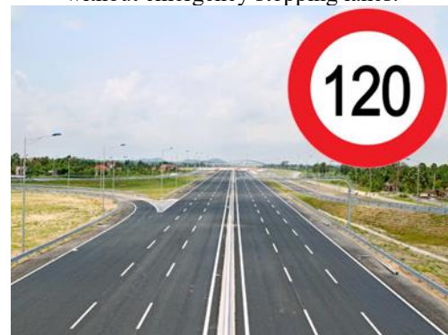
Full-phase expressway investment includes a 6×3.75m carriageway with a median barrier and 2×3m emergency stopping lanes
