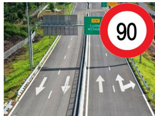
Initial-phase expressway investment includes a 4×3.5m carriageway with a median barrier but without emergency stopping lanes.
