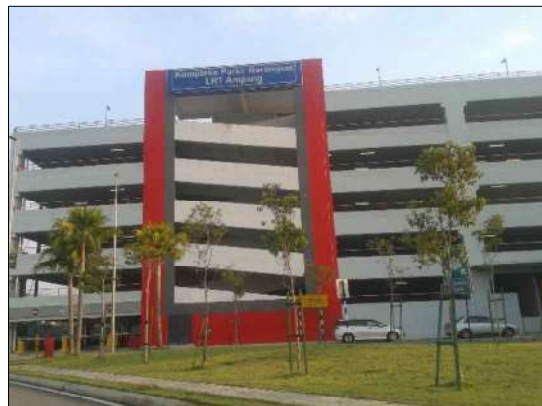
Figure 17. Park and Ride facilities
