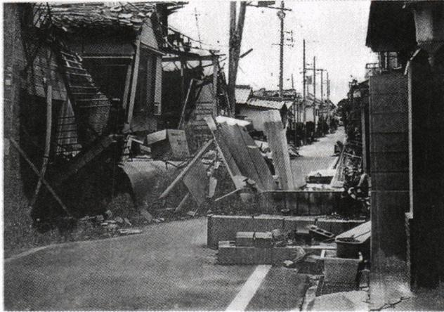
Photo 2. Residential Road Blocked by Topped Gate Poles and Chimneys (road width :6m)
