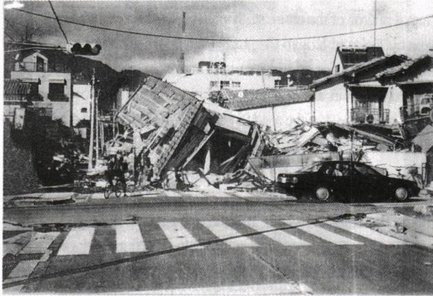
Photo 1. Local Distributor Road Blocked by Topped Houses (road width :12m)
