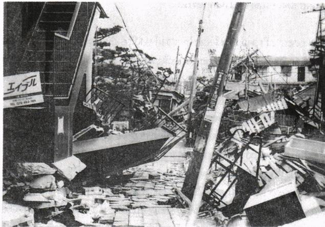
Photo 3. Residential Road Blocked by Topped Fences and Houses that Lined the Street (road width :4m)
