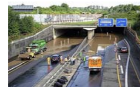
Inundation of tunnels
