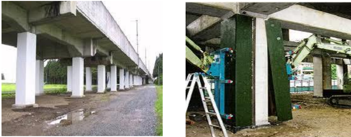
Figure 1. Viaduct Column Reinforcement
