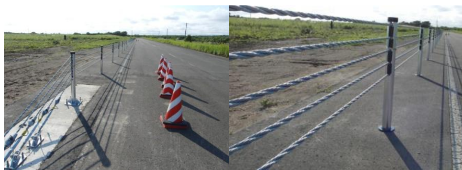
Figure 16. Guardrail after the second round of improvements
