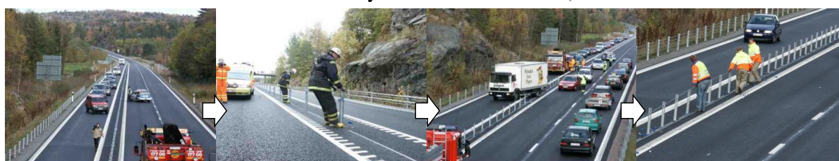
Figure 6. Median opening in emergency situations (from the Brifen website at http://www.brifen.co.uk/ )
