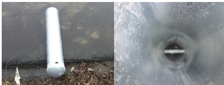
Figure 21. Sleeve and post support inside a pipe
