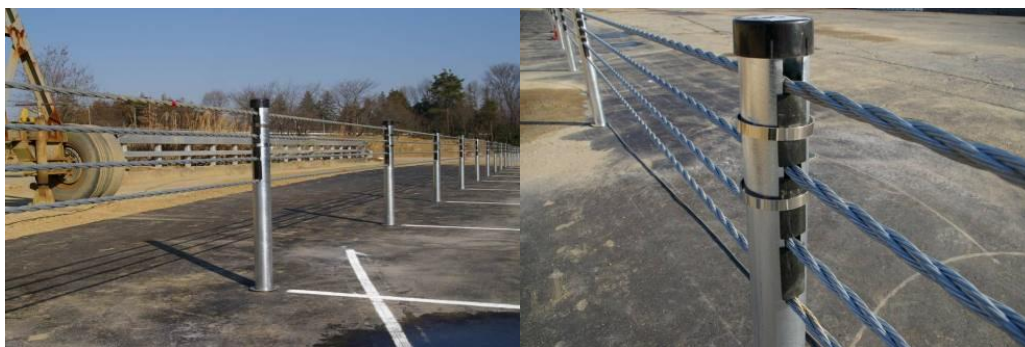
Figure 12. Improved wire rope guardrail system
