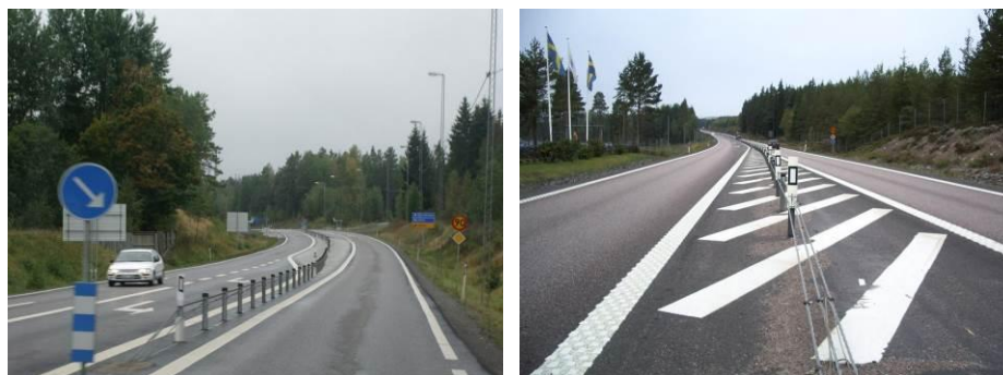
Figure 3. 2 + 1-lane road with a wire rope guardrail system (Sweden)
