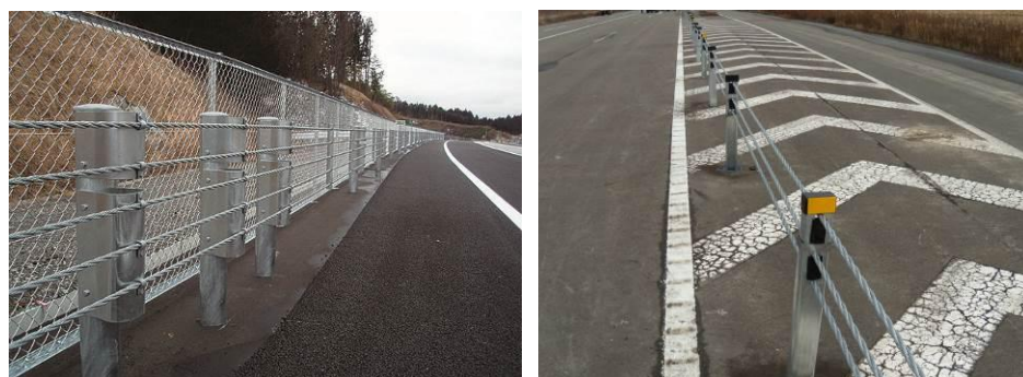
Figure 4. Guard cable (left) and wire rope (right) guardrail system
