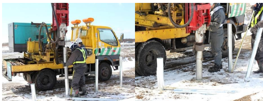
Figure 23. Sleeve placement
