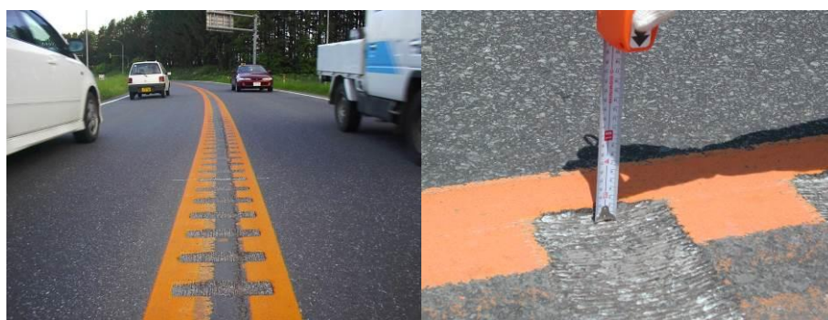
Figure 2. Centerline rumble strips (left: R237; right: R275)
