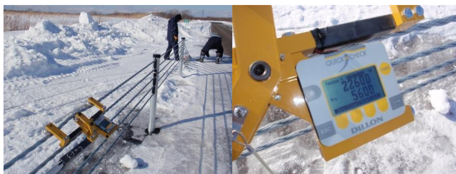
Figure 24. Stretching and tension measurement
