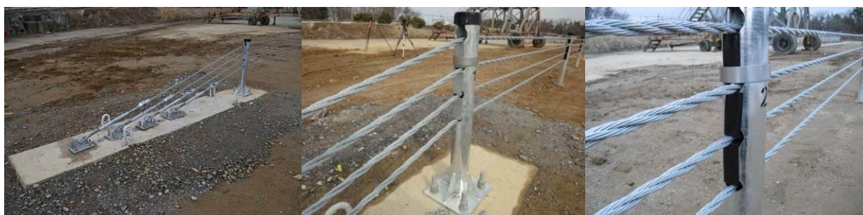
Figure 10. New wire rope guardrail system
