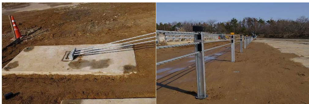
Figure 8. Wire rope guardrail system of Trinity Industries, Inc.
