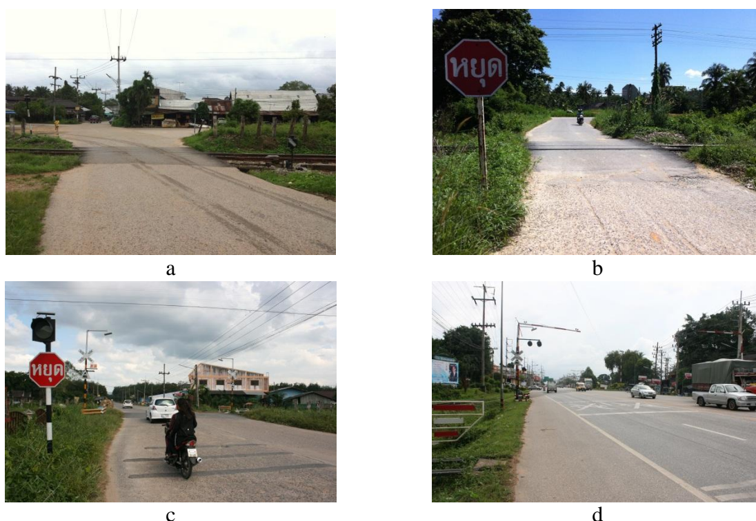
Figure 3. (a) Illegal; (b) Stop signs; (c) Flashing lights; and (d) Half lifting barriers
