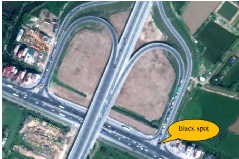
Figure 17. The 4 th black spot (B4): The Fork - section of NH 5 at Km 6
