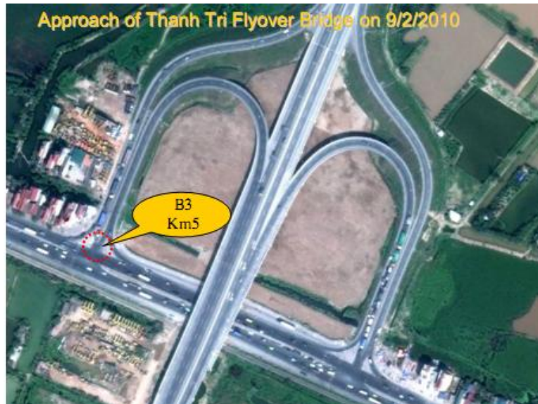
Figure 15. The 3 rd black spot (B3): The fork-section of the NH5 at Km5
