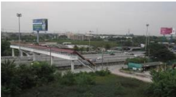
Pedestrian bridge above the Motorway
