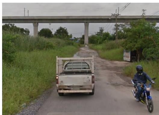
Road condition at the end of Chaloei Phra Kiat Ratchakan Thi 9 road
