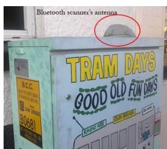
Figure 4: Scanner antenna on top of the signal controlled box. The scanner is installed in the in the signal controller (Brisbane, Australia)
