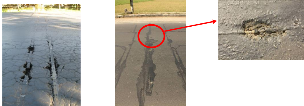
Figure 6. Damaged sensors
