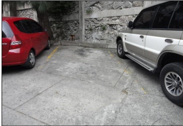
Figure 12. Faded parking guide markings
