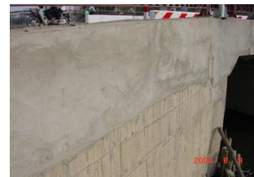
Poor surface finish
