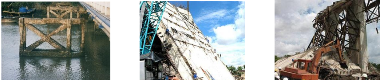
Figure 2. Failure of existing concrete bridges
