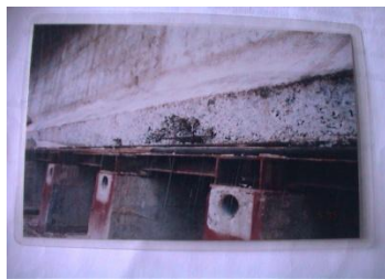
Concrete honeycomb
