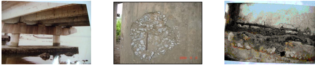
Figure 4. Damage of existing concrete bridges in Vietnam
