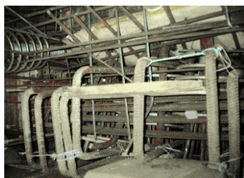
Over-density of rebar
