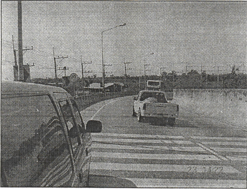
Figure 3. The Driver Changing from the Inner to the Outer Lane Could Cause a Side Collision.
