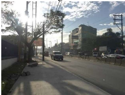
Figure 1. Road Section S01598LZ - Photographed on Feb. 26, 2018
