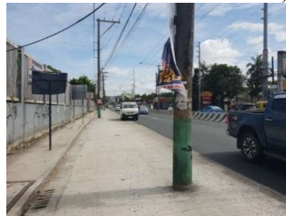
Figure 2. Road Section S01598LZ - Photographed on Jan. 20, 2019
