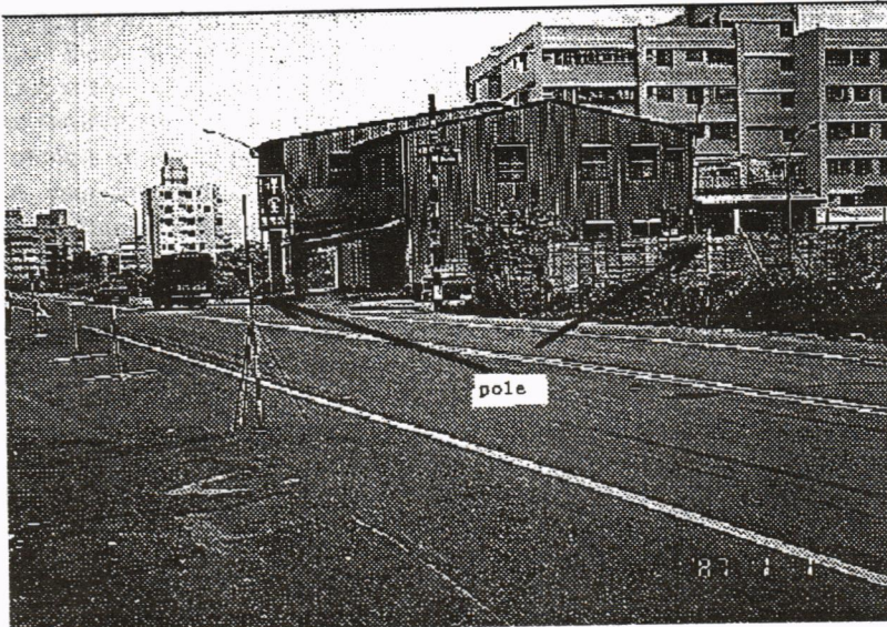
Figure 6 Poles setting along the roadside .
