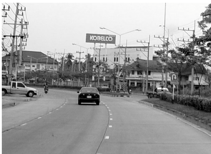
Figure 5. U - turn opening without a storage lane creates potential for rear end collisions.
