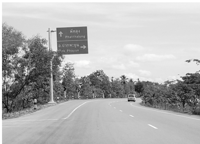
Figure 3. Large pole located on curve poses a potential hazard.
